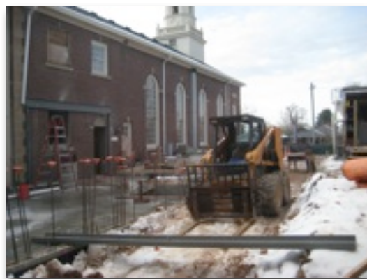
Photo of construction progress as of January 30, 2012.
